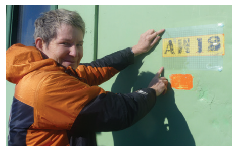
Conservator Sue Bassett carefully stripped back layers of paint to reveal some of the original stencilling used to identify the different panels of the pre-fabricated Scott Base. © AHT
