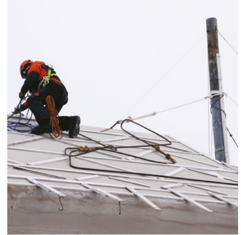
Replacing the anchoring rigging on Shackleton's Hut at Cape Royds. ©AHT/Lizzie Meek
