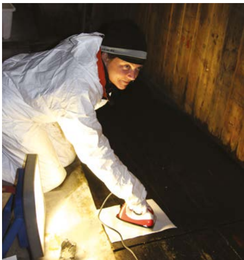
Conservator Jane Hamill removes the residual blubber oil by drawing it out into blotter paper with the heat from a ski-waxing iron, in Scott's 'Discovery' hut. © AHT/AI Fastier
