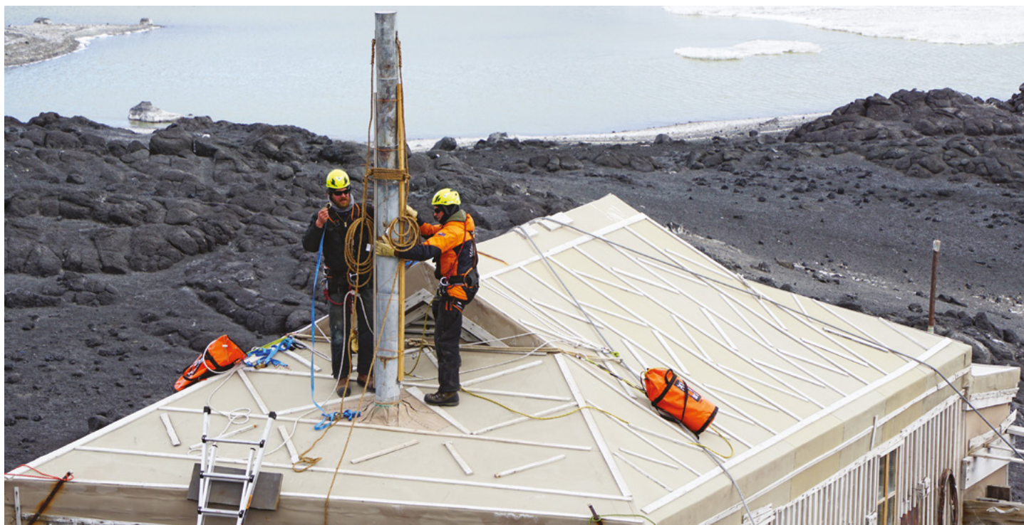
L-R: Zack Bennett and Lachie Cromar reinstate the chimney flue on top of Shackleton's 'Nimrod' hut. © AHT/Jane Hamill
