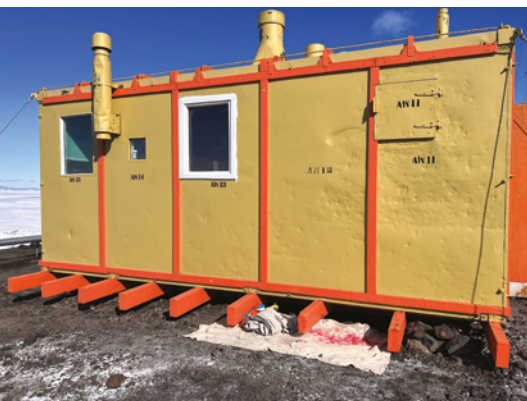
Painting underway on Hillary's TAE/IGY hut. © AHT/Zack Bennett
