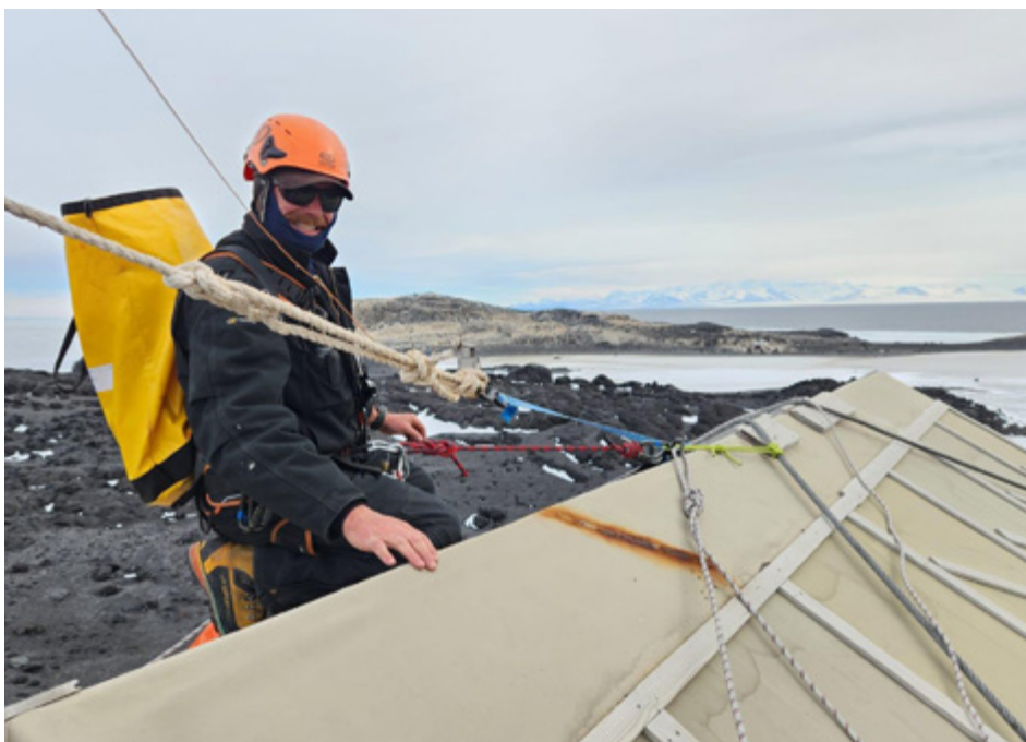
Building Conservation Programme Manager Zack Bennett repairing a rigging anchor on the roof of Shackleton’s Nimrod Hut © AHT/Johan Bergman
