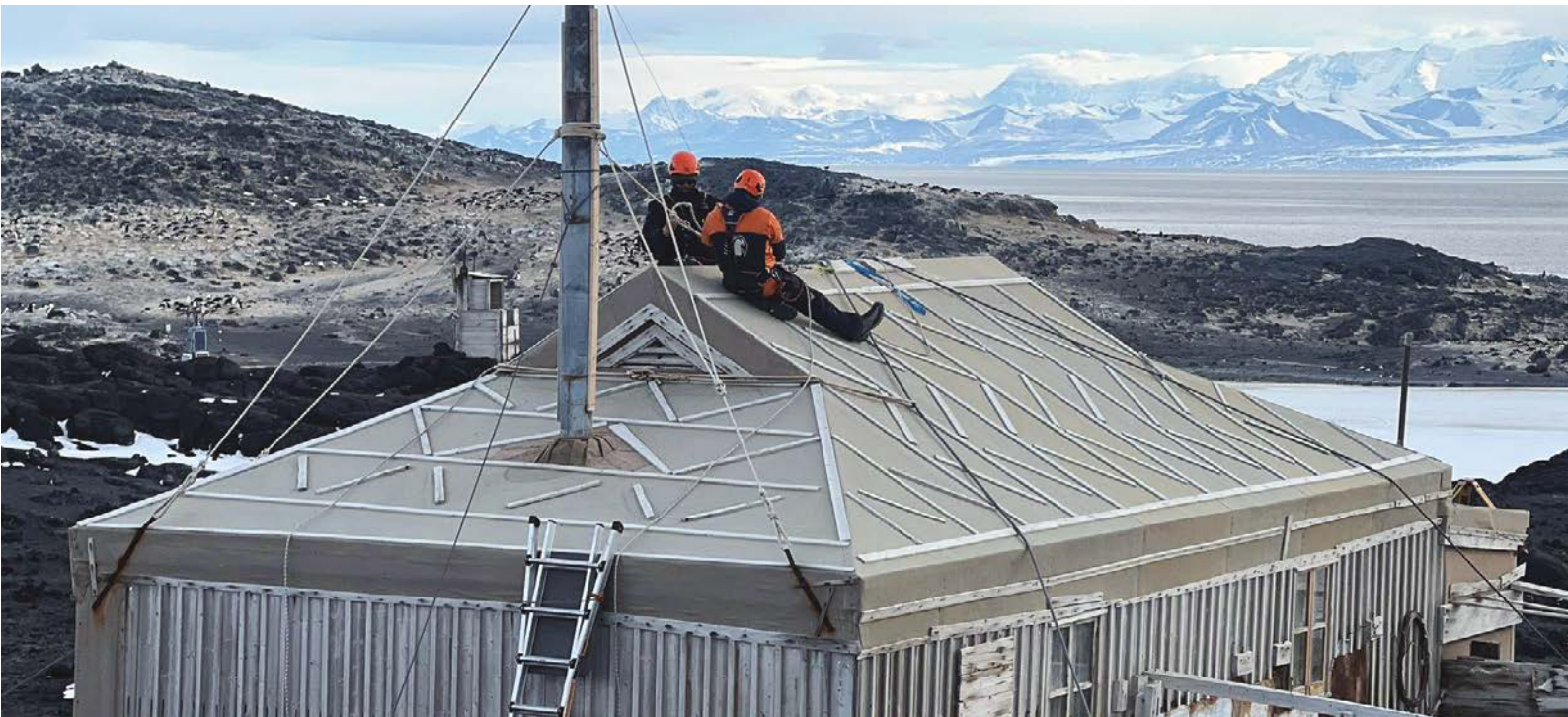
Building Conservation Programme Manager Zack Bennett and GM Programmes Johan Bergman, undertaking chimney fitting repair to Shackleton's Nimrod hut at Cape Royds. © AHT/Jeremy Moyle
