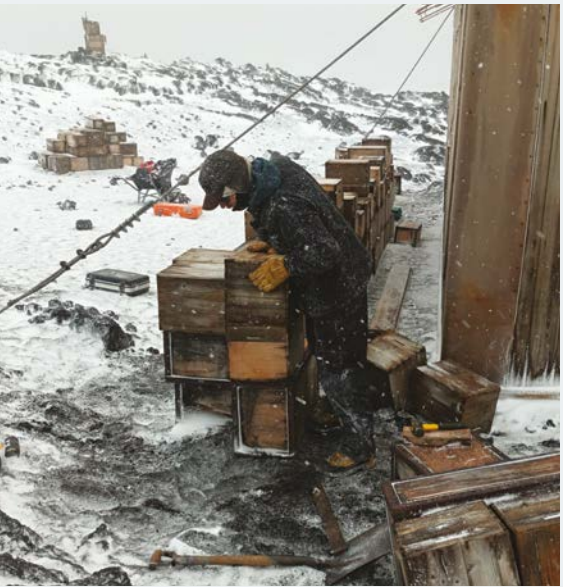
STORM DAMAGE REPAIRED
